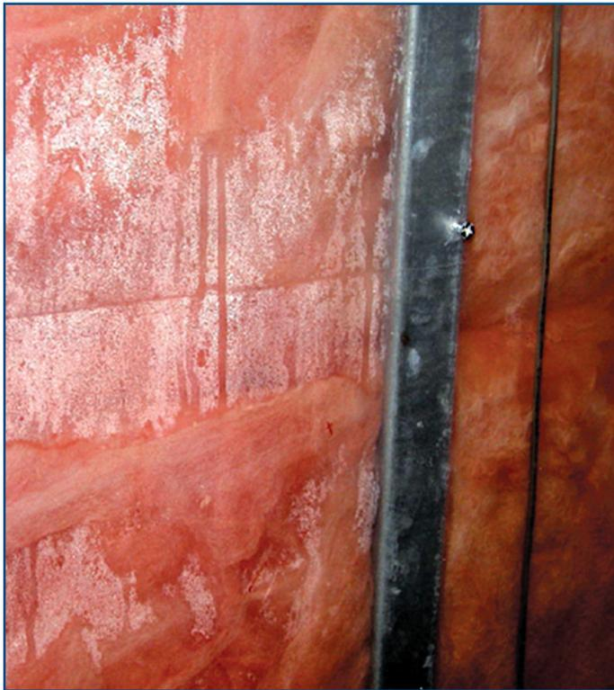
Figure 6 – Example of inward vapor driven condensation on the cooler interior vapor barrier.
